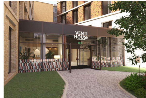
Venti House, Stratford - PBSA
